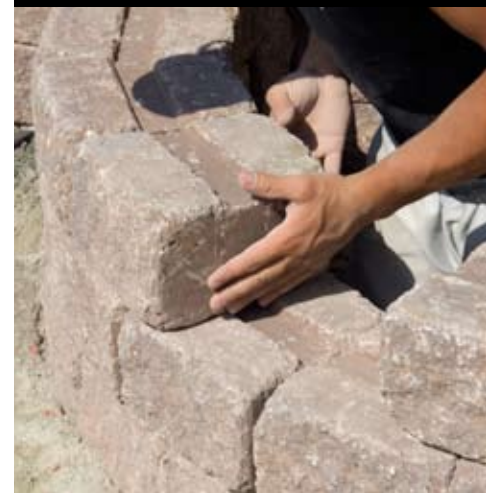
THE FORTRESS BLOCK CONNECTOR LETS YOU PLACE LOW WALLS IN STRAIGHT LINES, CURVED LINES OR IN STAIRCASE FORMATIONS.
