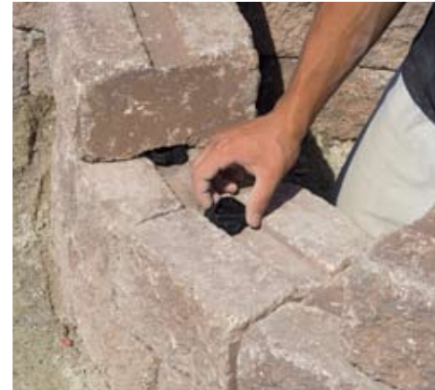
THE FORTRESS BLOCK CONNECTOR LETS YOU PLACE LOW WALLS IN STRAIGHT LINES, CURVED LINES OR IN STAIRCASE FORMATIONS.
